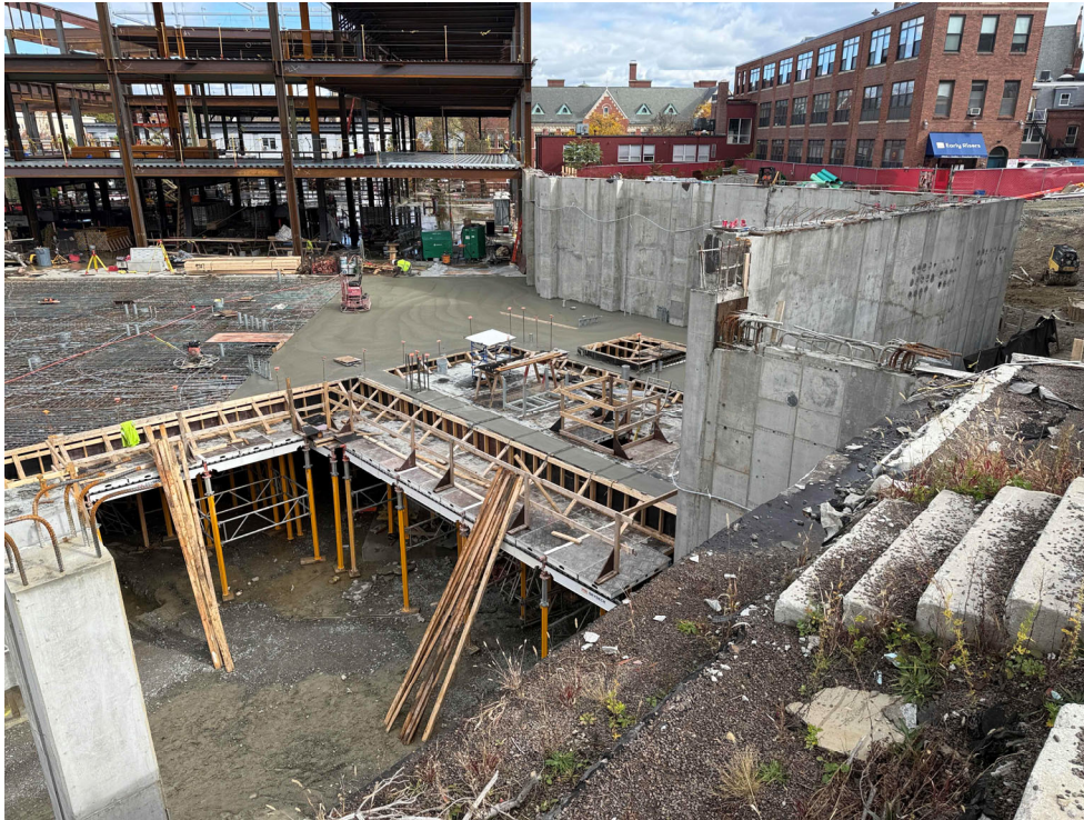
Building B structural deck concrete placement #5, 10/31
