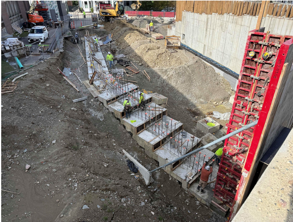
Retaining wall footing, 10/15
