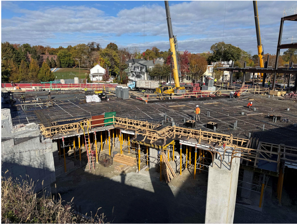
Building B structural deck: rebar, sleeves, formwork, 10/27
