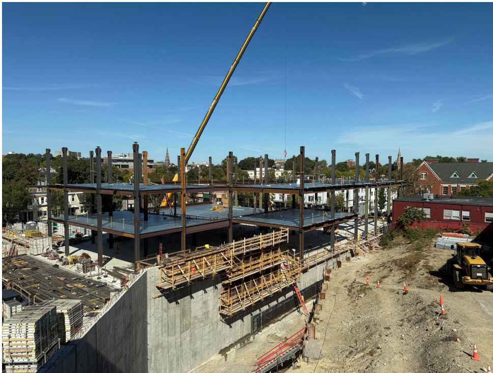
Steel frame progress, 10/03
