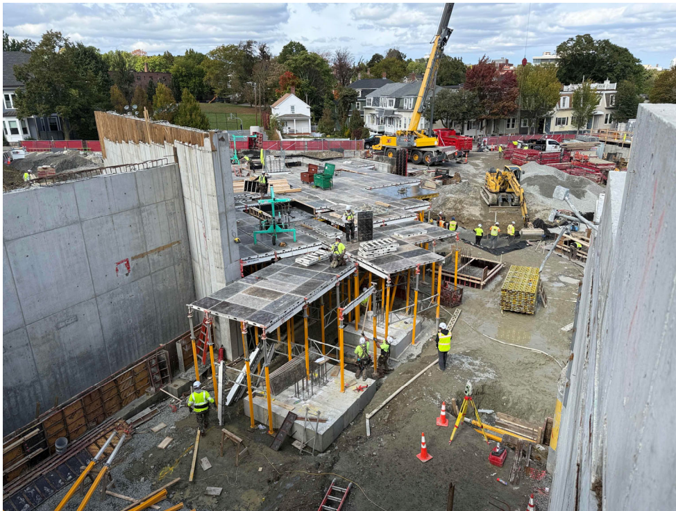
Building B structural deck, 10/15
