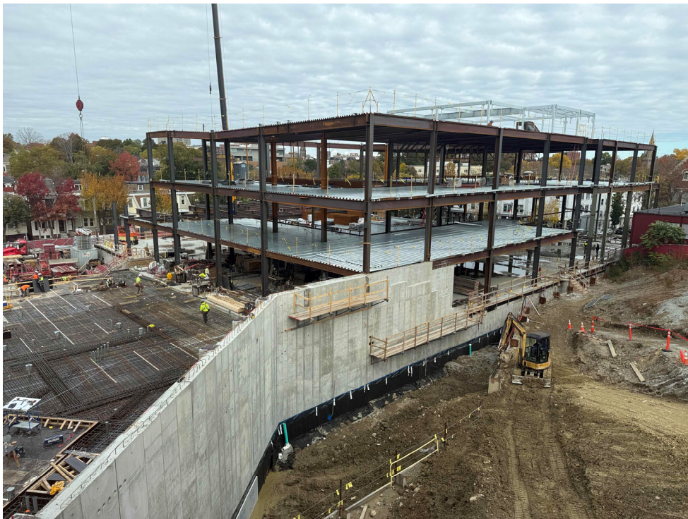
Steel frame progress, 10/24
